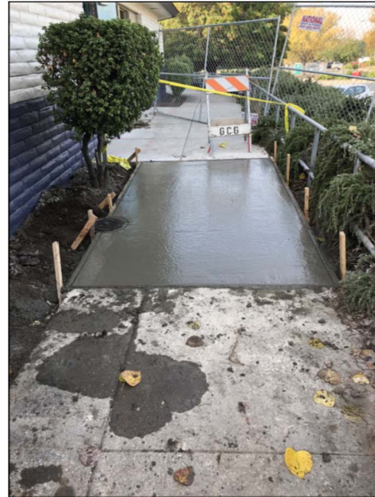
ADA upgrades to path of travel
