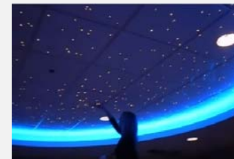
Acoustic panels with fiber optics as the night sky
